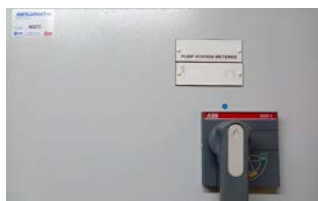
Switching Mechanism to enable Fujitsu Datacenter UPS to power local water pumps in the event of a flood (United Kingdom)
