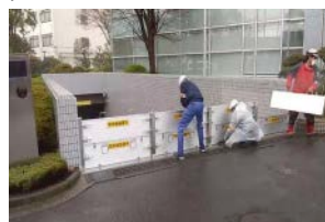
(a) Removable watertight panels
