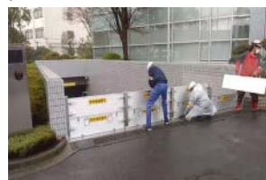
(a) Removable watertight panels
